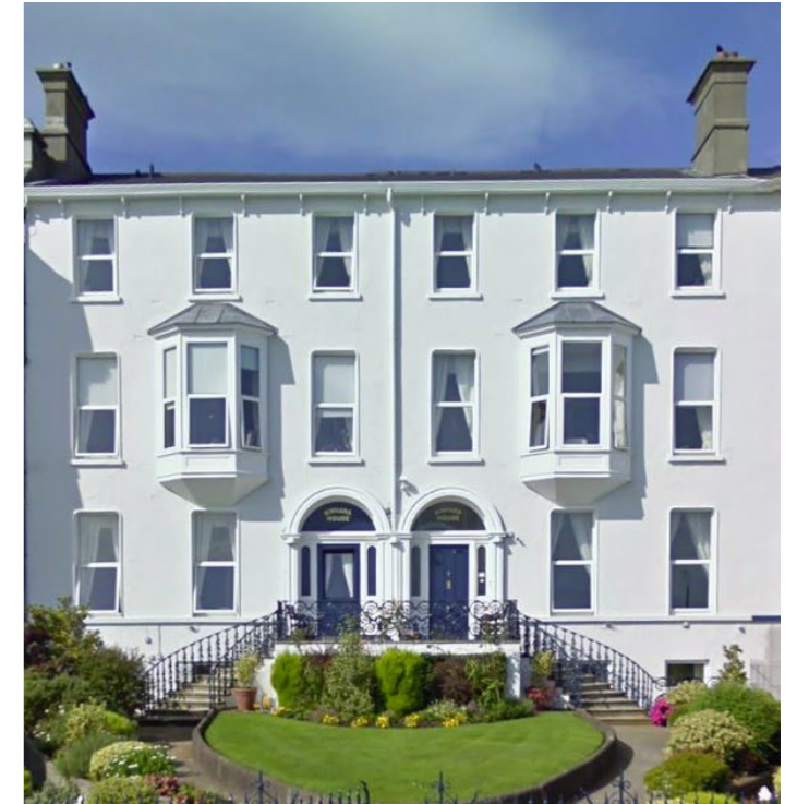
Promenade Terrace with Large Bay windows
